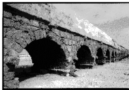
A Roman aqueduct
